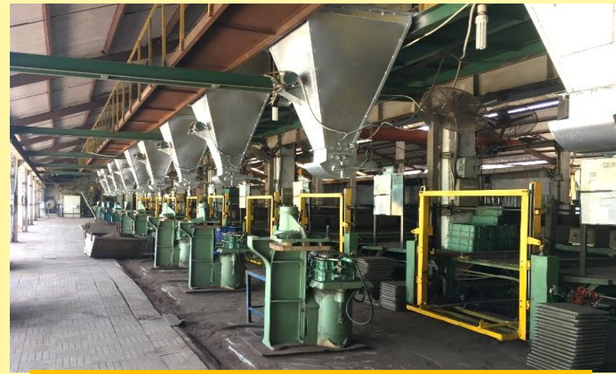
CASTING (7.200 tons/ year)
